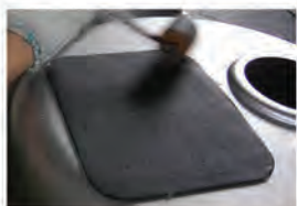
When applying the pad to the sink, a roller is used to flatten or even out the pad.
